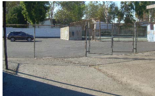
Major improvements are needed in security fencing.
