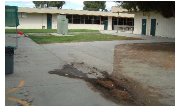
Poor concrete/asphalt conditions campus wide.
