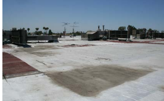
Replace roofing and HVAC units.
