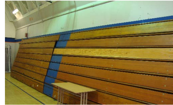
Need to replace gym bleachers.
