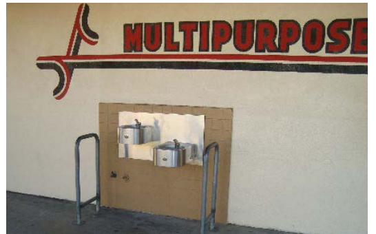
Interior/exterior of buildings need to be repainted.
