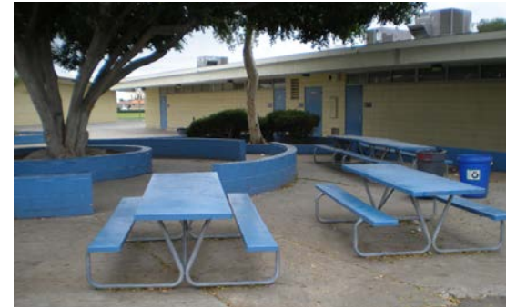
Need lunch shelters throughout campus.
