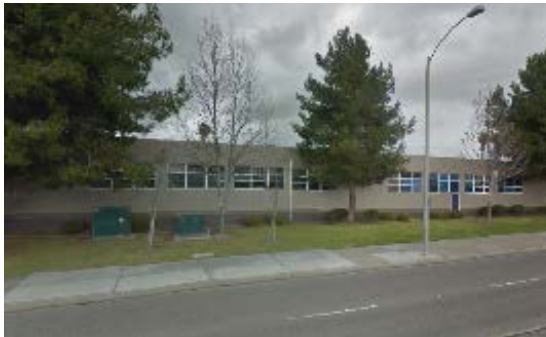
Campus in vital need of fencing/security improvements
