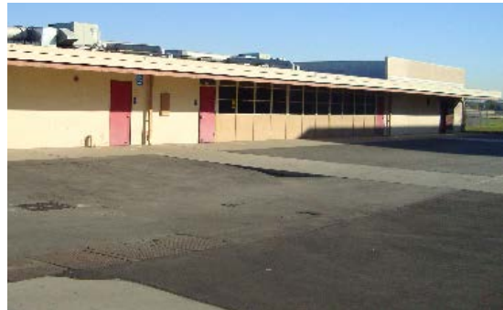
Existing paving in poor condition throughout campus.
