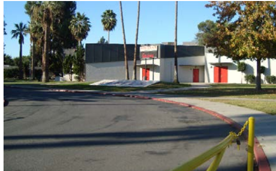
Major improvements needed to drop off and parking areas.
