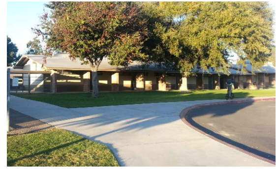
Need to reconfigure campus entry/exit.
