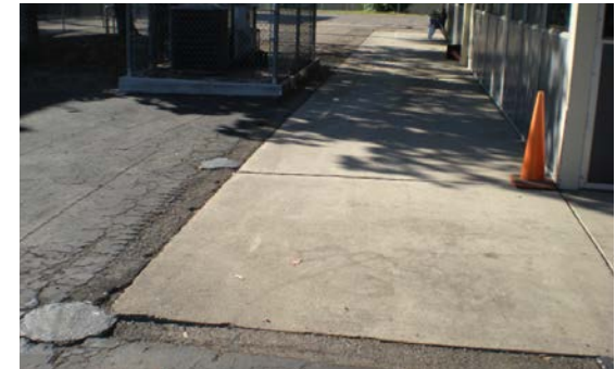
Paving in poor condition across campus.
