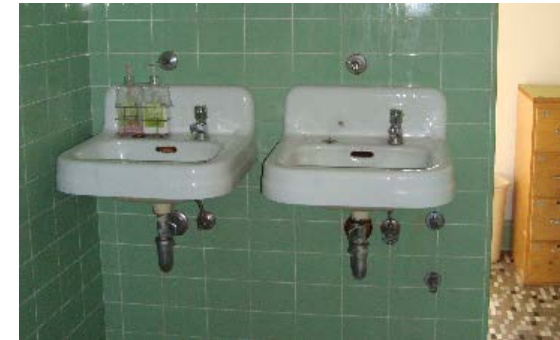
Restrooms are in need of upgrades.
