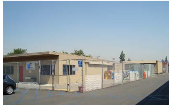
Replace relocatable buildings with permanent construction.
