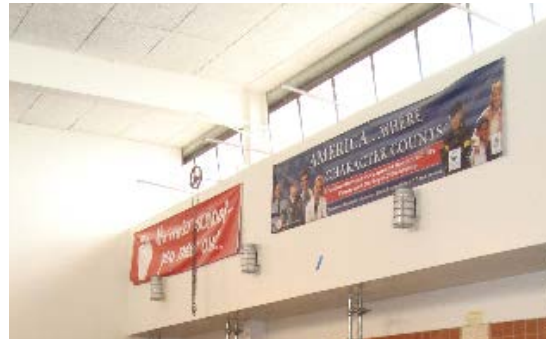
Replace leaking clerestory windows in locker rooms.
