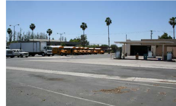
Slurry seal fueling station.
