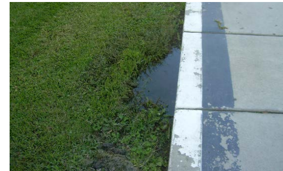
Address flooding/ponding issues between buildings.
