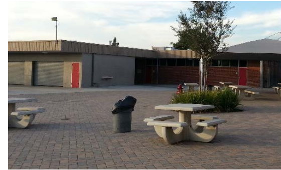
Need new shade structures/lunch shelters.
