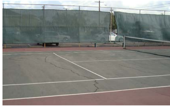
The tennis courts need to be replaced.
