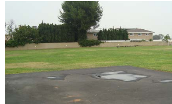
Minor ponding and flooding issues on campus.
