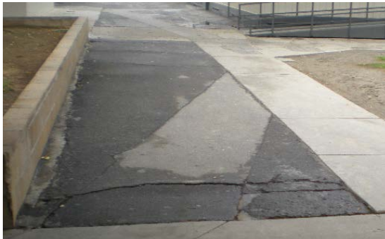
Campus wide asphalt paving in poor condition.
