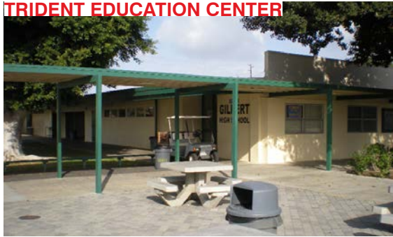
Shade structures are needed.
