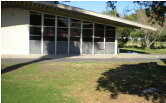
Landscape and irrigation in need of renovation.
