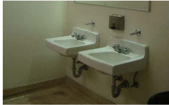
All restrooms need renovation.
