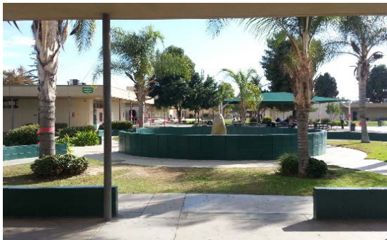
The campus quad needs lunch shelters/ADA accessibility and improved drainage.
