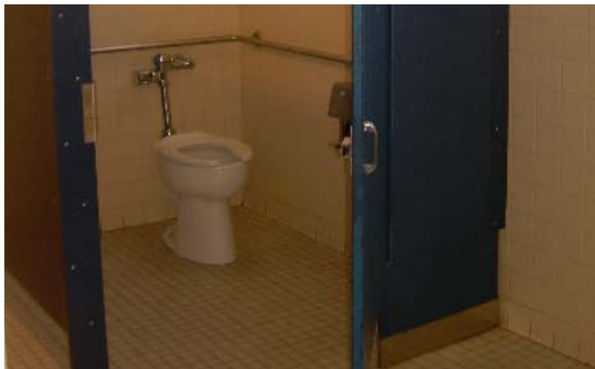
Upgrade and expand restroom facilities.
