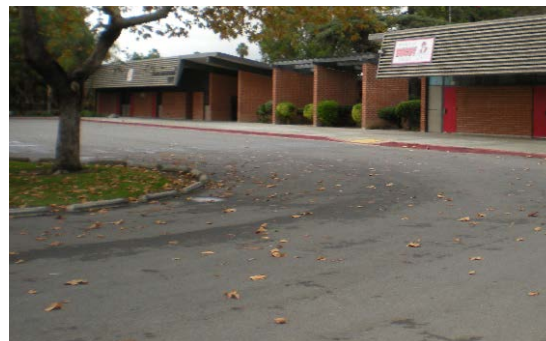
Improve parking and drop off.
