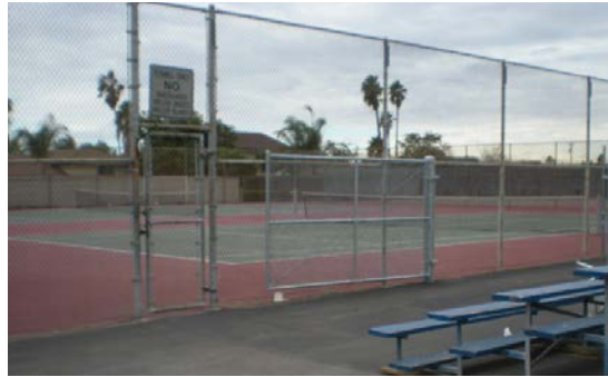
Need to refurbish tennis courts.
