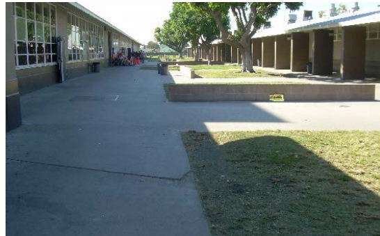
Overall paving in poor condition across campus.
