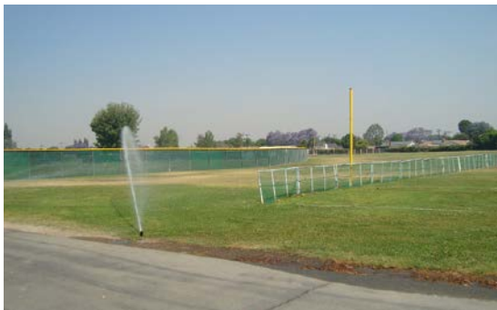
The athletic fields need new irrigation system.
