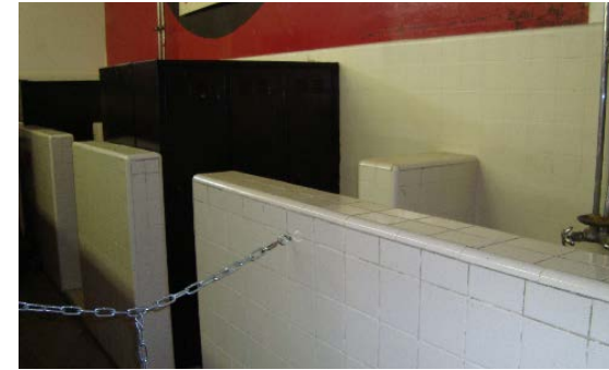
Locker rooms in need of expansion/consolidation.
