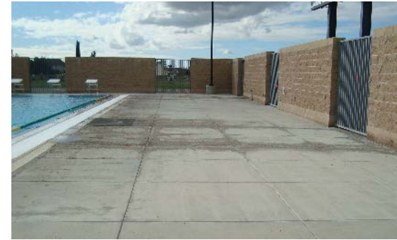
Pool in need of modernization; deck resurfacing.
