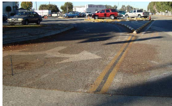
Reconfigure and upgrade main parking lot.
