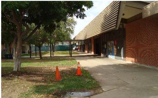
Major drainage/ponding issues in campus courtyards.
