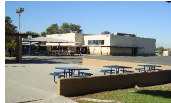
Lunch shelters need to be replaced/expanded.
