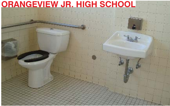
Campus restrooms are in need of an upgrade.
