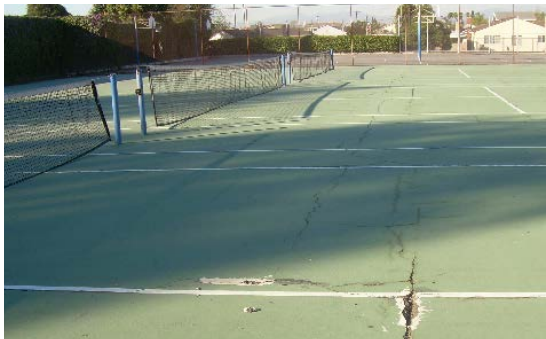
Tennis courts require resurfacing and/or replacing.
