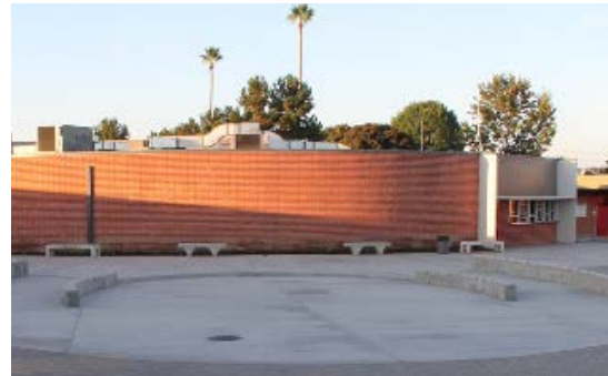
Loara Theater in need of upgrades.
