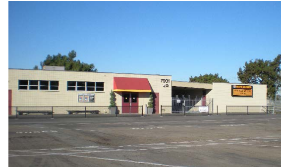
Need to improve drop-off/bottleneck for wheelchairs.
