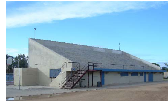
Replace concrete bleachers.
